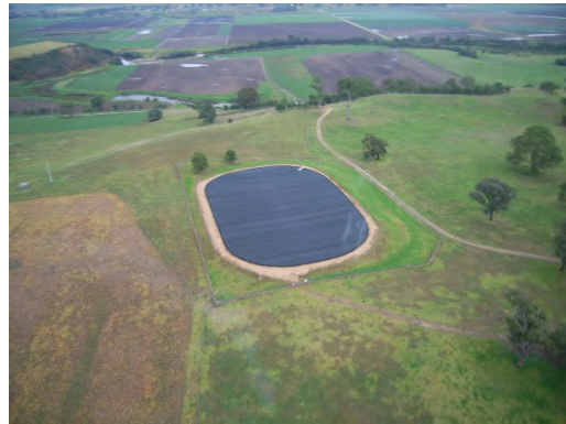
Figure 16: Lindenow clear water basin
